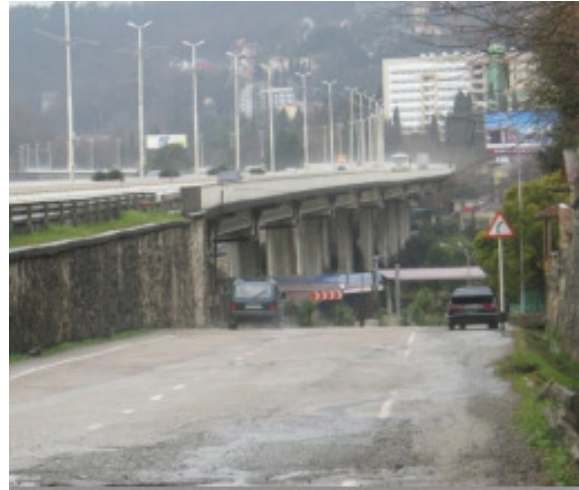
Fig. 3. Electric lighting of roadway on the bridge
